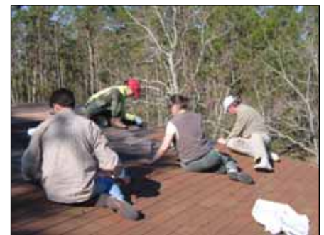
Roof repair crew
