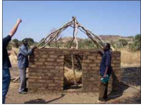
A student mud-brick hut under construction.
